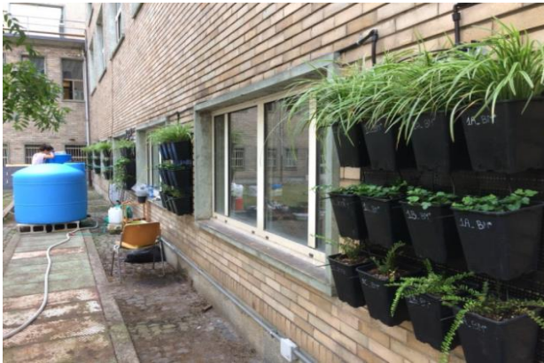
Figure 1. Pilot system installed in the courtyard of the laboratory.
